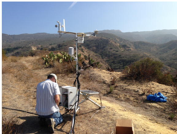
Figure 2 – An example weather station. The towers are less than 3.5 meters in height, contain equipment on side-arms, and can be painted to avoid contrasts with the landscape and reduce their view-shed impact.
